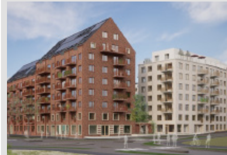
MTA is constructing the first phase of a new residential development in Västerbro, Lund, on behalf of Huseriet/Rikshem. Västerbro is one of Lund's oldest industrial areas.
