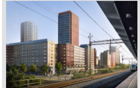
K-Prefab has delivered a complete structural frame contract for the development of residential units, commercial premises and a parking garage in Årstaberget, Stockholm, for the client Nocon. Early concept illustration of the planned development. Architect: FOJAB
