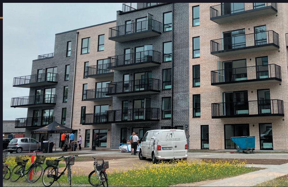
Emilienhaven in Vallensbaek. Our first in-house project in Denmark where tenants are moving in under phase one in June 2022.
